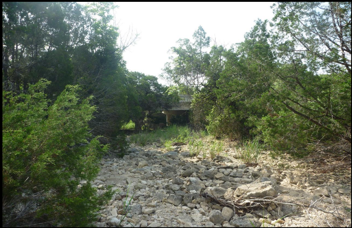
Photo 3. West of Slaughter Creek Bridge, looking east
